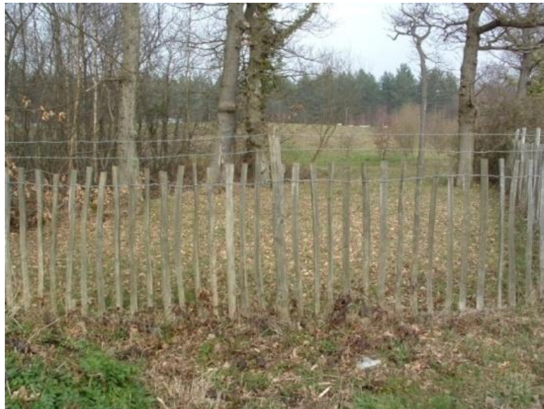
Figure 4.5 Pale fencing, with a top wire
