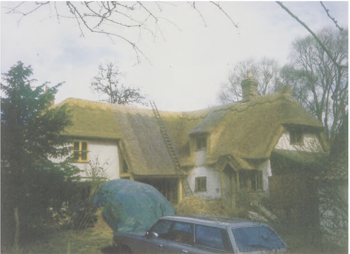
Illustration 6 - Block cut ridge in water reed at Riddy Lane, Bourne (Bo 01).
