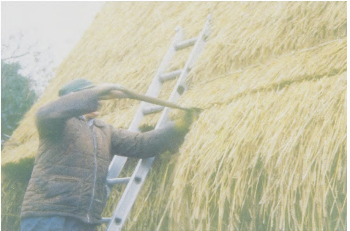
Illustration 12 - Long wheat straw roof with eaves being cut to shape (centre and left of ladder), with waste straw still in place before being trimmed off
