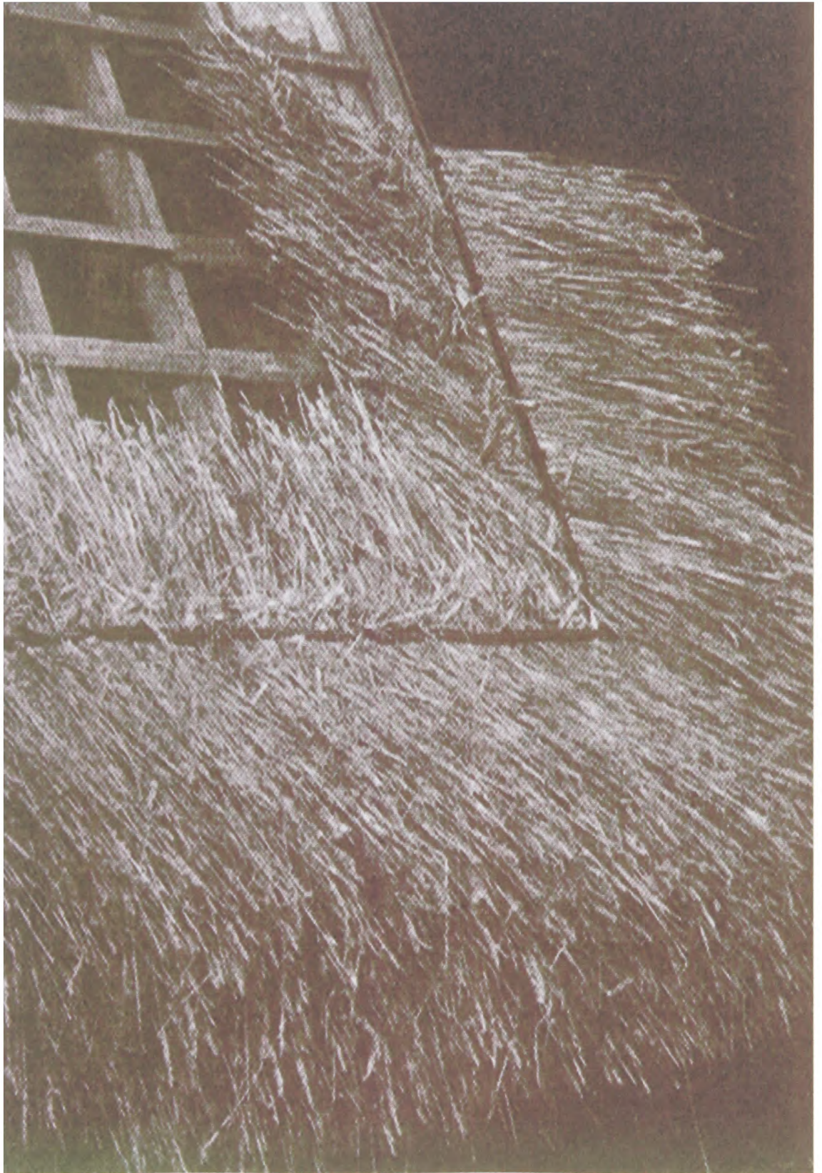
Illustration 29 - Bottles secured along the eaves and barge
