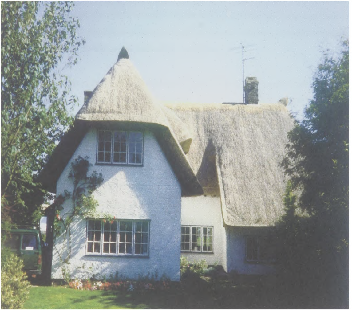
Illustration 16 - A newly thatched long wheat straw roof at The West Green, High Street, Barrington (Ba 03), showing how the straw seems to have been poured over the bones of the structure
