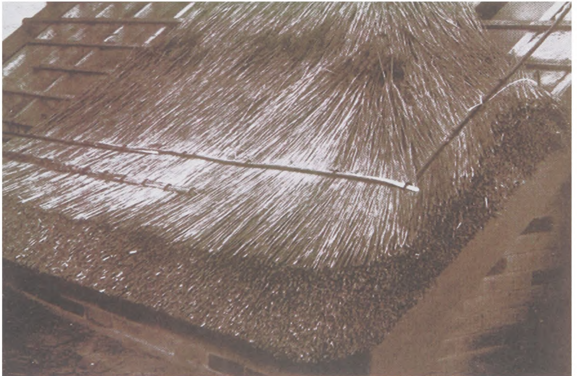
Illustration 67 - A full course with sway fixed with tarred cord
