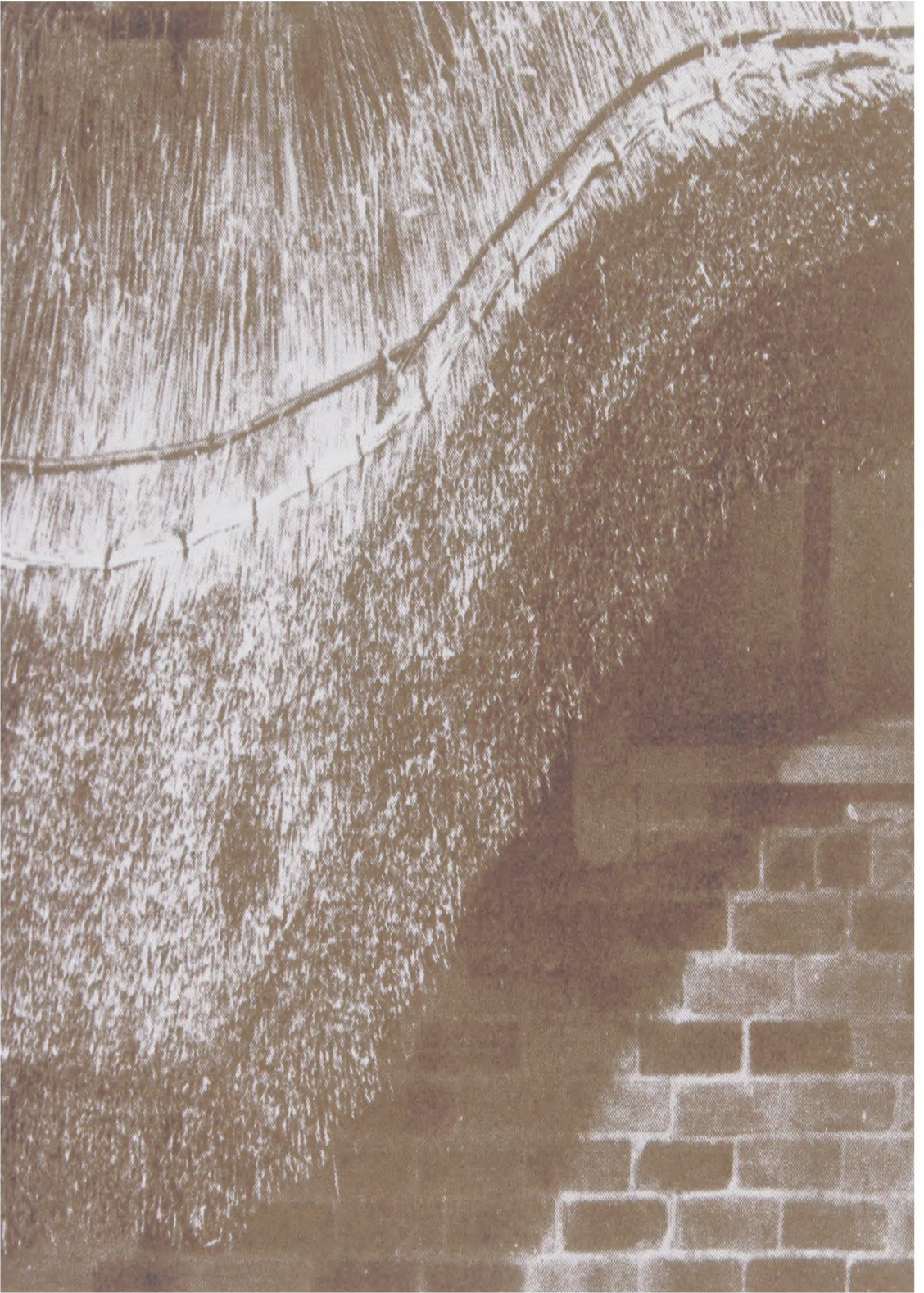
Illustration 48 – The relationship of the sways to an eyebrow (with a temporary straw sway still in position just beneath)
