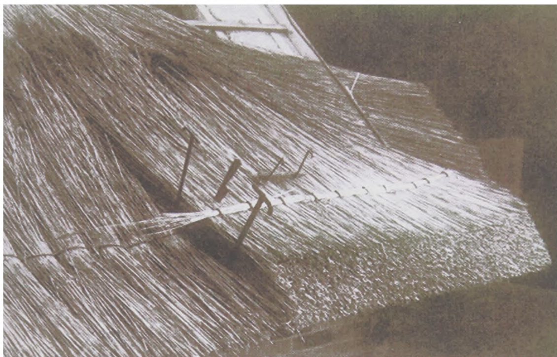
Illustration 62 - A brow course fixed with temporary sways and hooks
