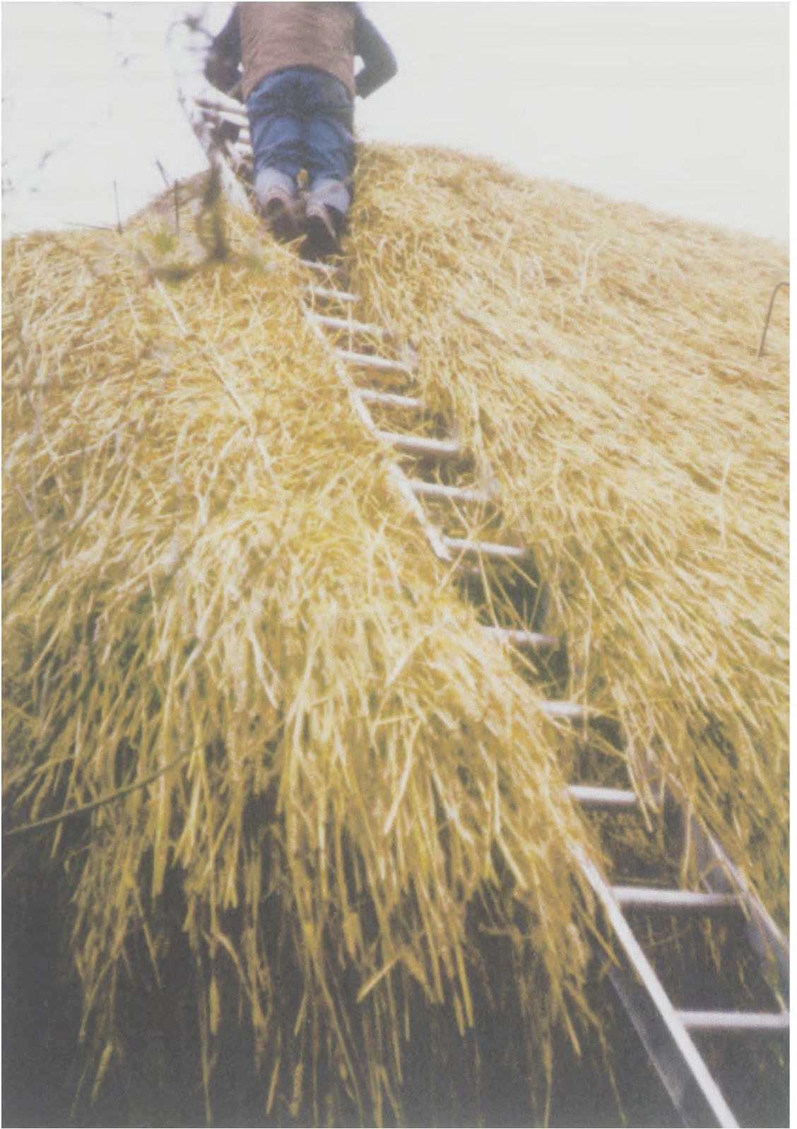
Illustration 37 - Completed left barge course, with the ladder course still to be completed
