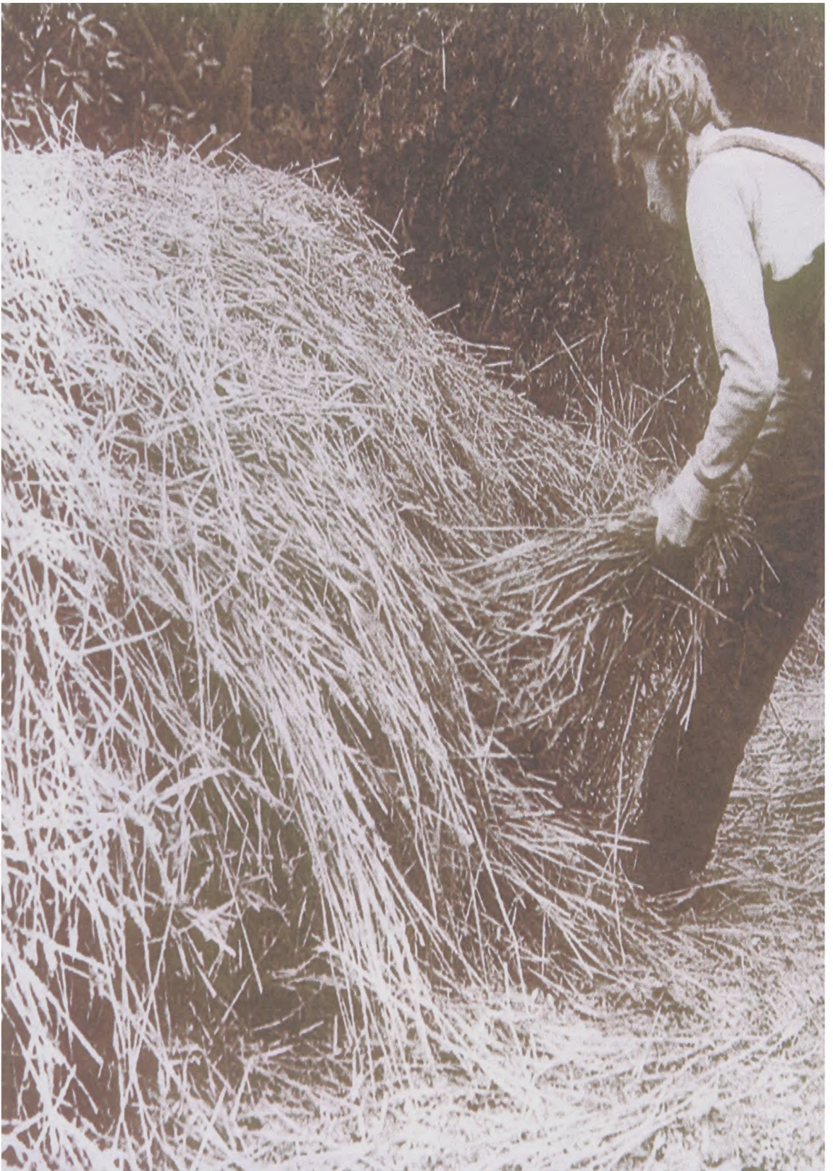
Illustration 20 - A master thatcher drawing straw from a bed to form a yealm
