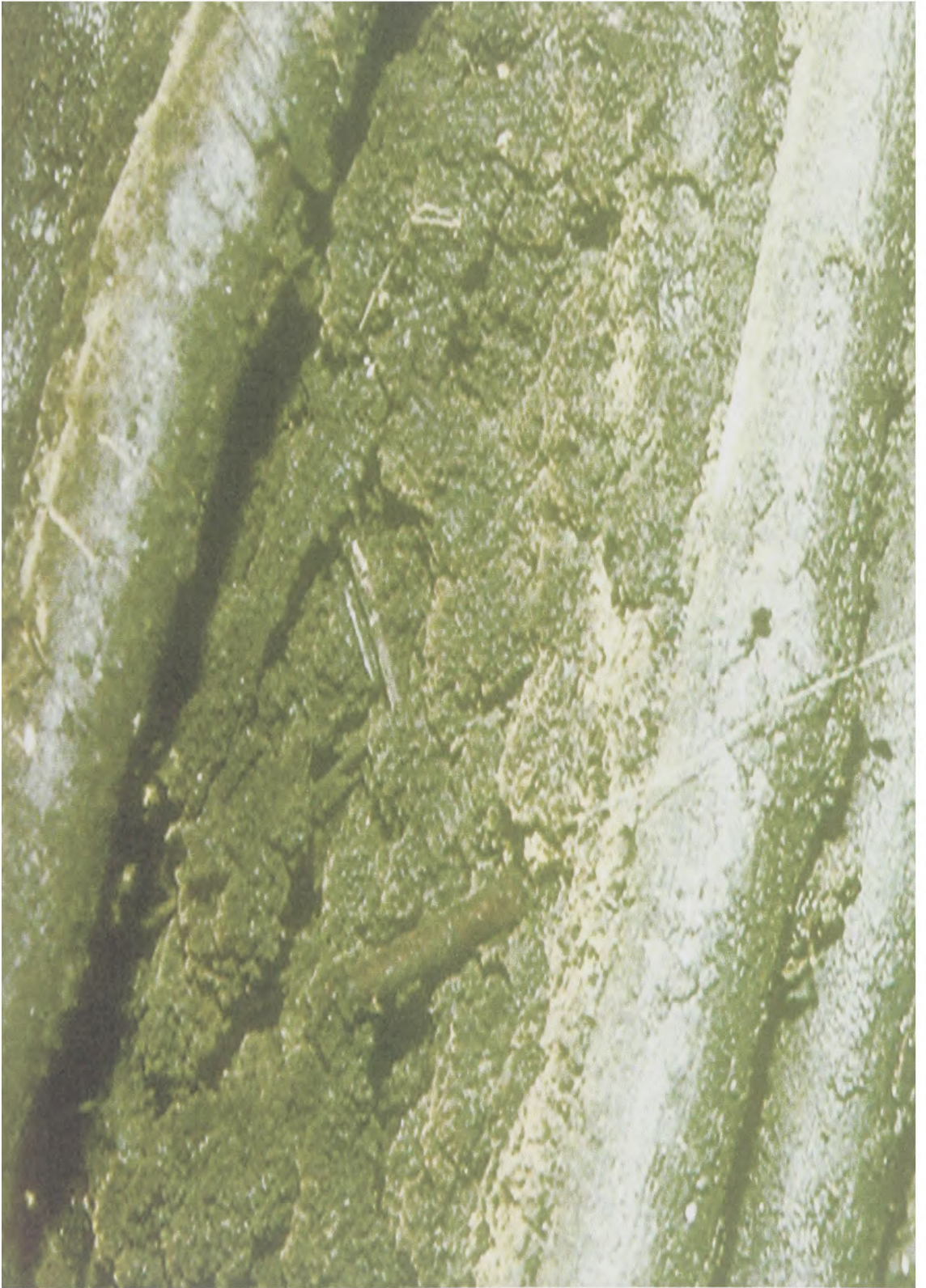
Illustration 68 - A formation of smoke-blackened thatch
