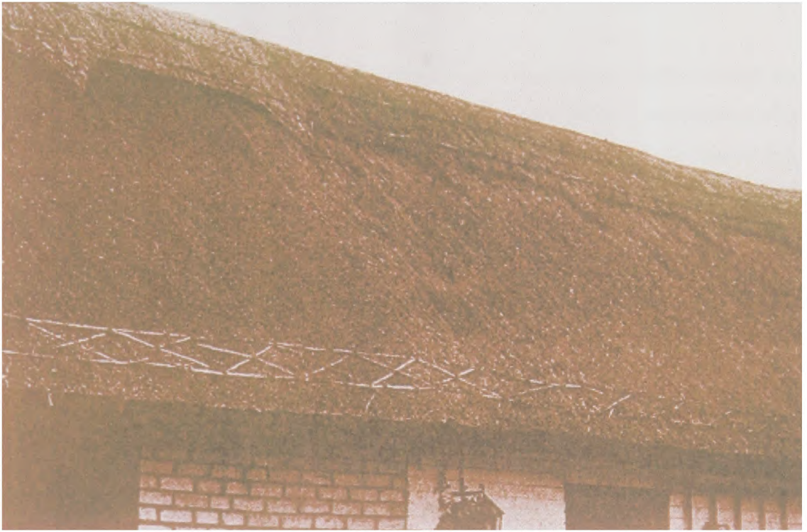
Illustration 9 - Liggers on a long wheat straw roof, extended in combed wheat reed
