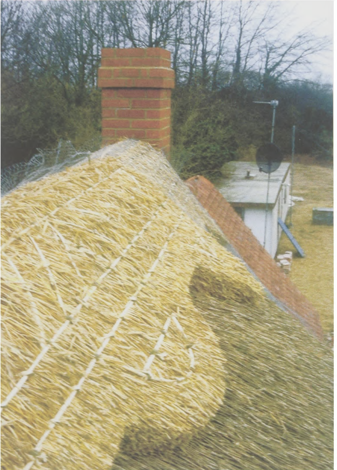
Illustration 7 - Block cut ridge in long wheat straw at 41 Whitecroft Road, Meldreth (Me 02)
