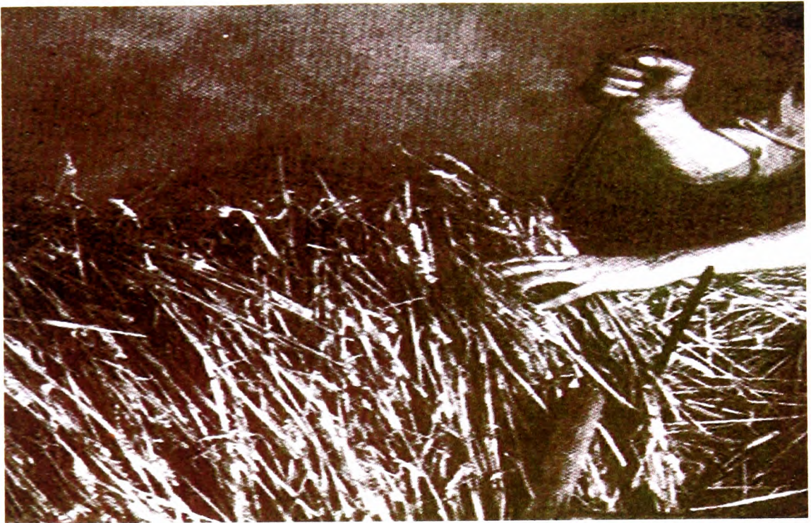
Illustration 40 - Needles being used in order to compress the additional thatching straw
