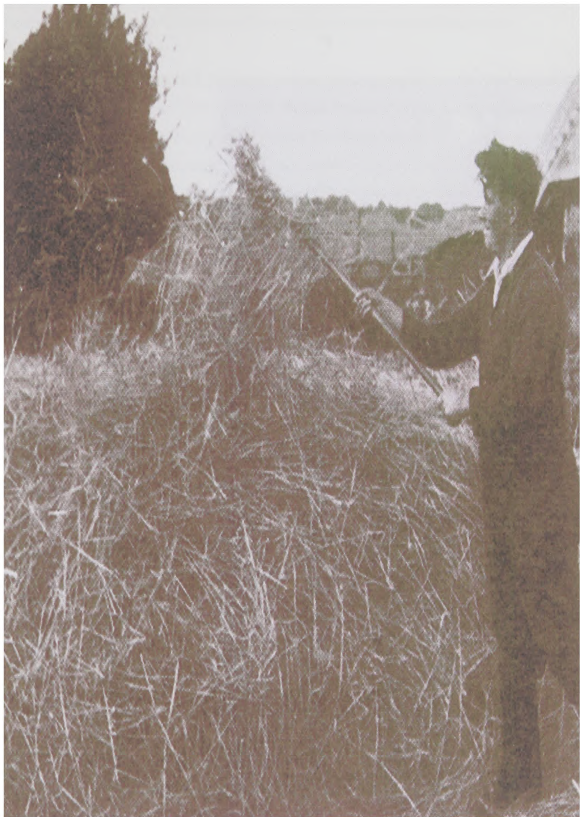
Illustration 19 - Straw shaken into a heap forming a bed from which the yealms are drawn
