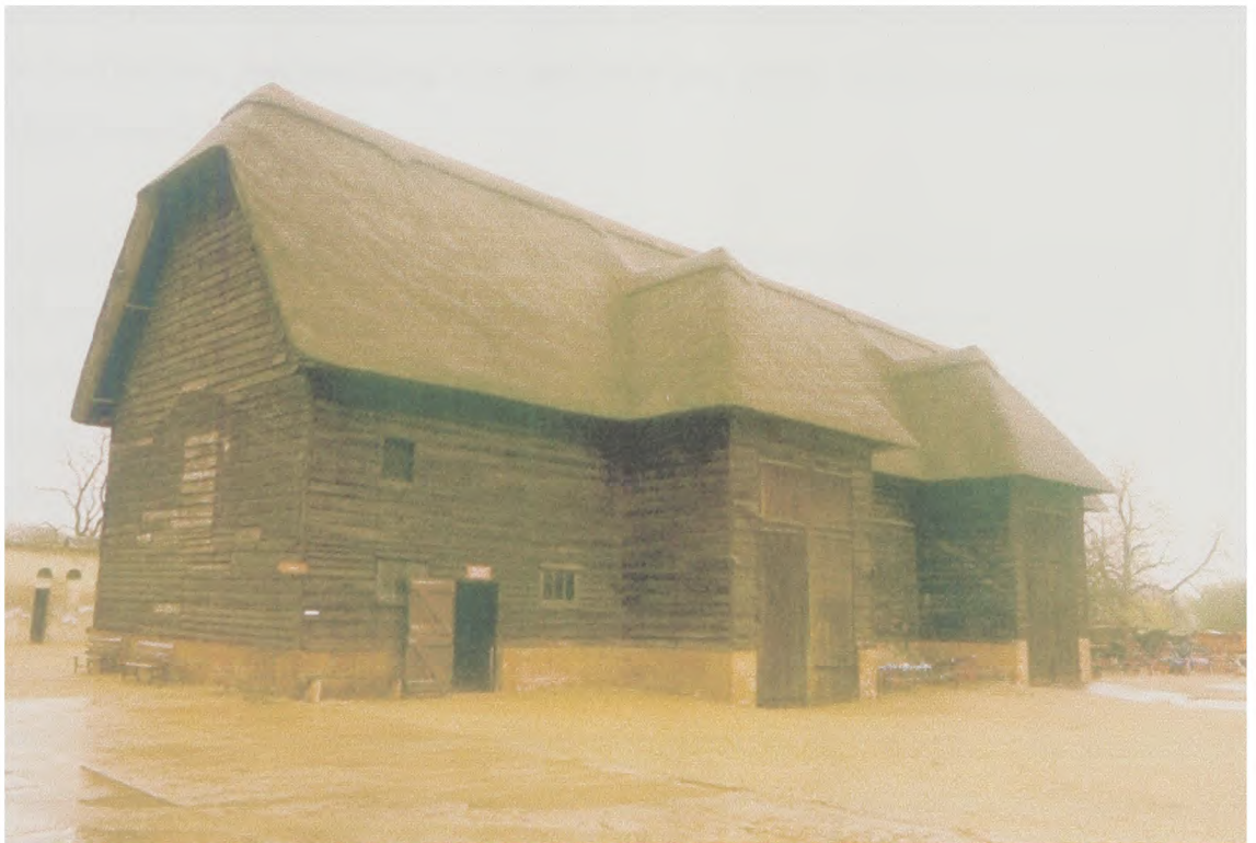
Illustration 4 - Water reed thatch on the roof of the Great Barn at Wimpole (Wm 01)
