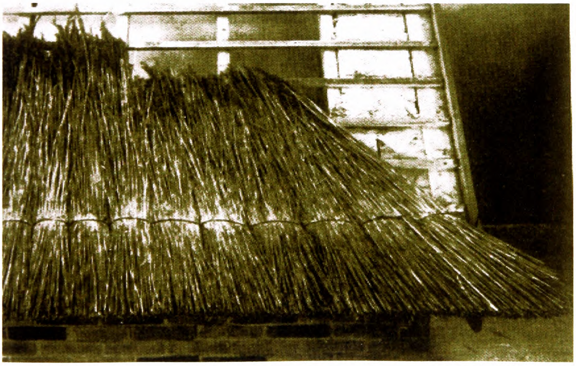
Illustration 60 - Direction of the wadds
