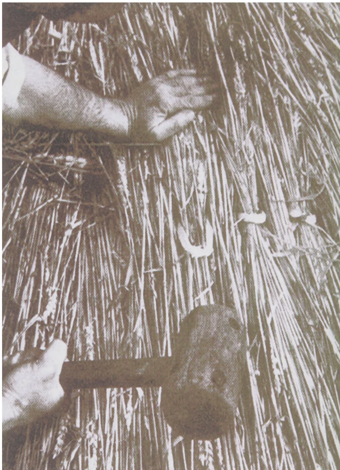
Illustration 34 - An extra yealm laid to a corner, showing the row of spars halfway between the hammer and the thatcher's left hand, and the tarred cord immediately below his left hand
