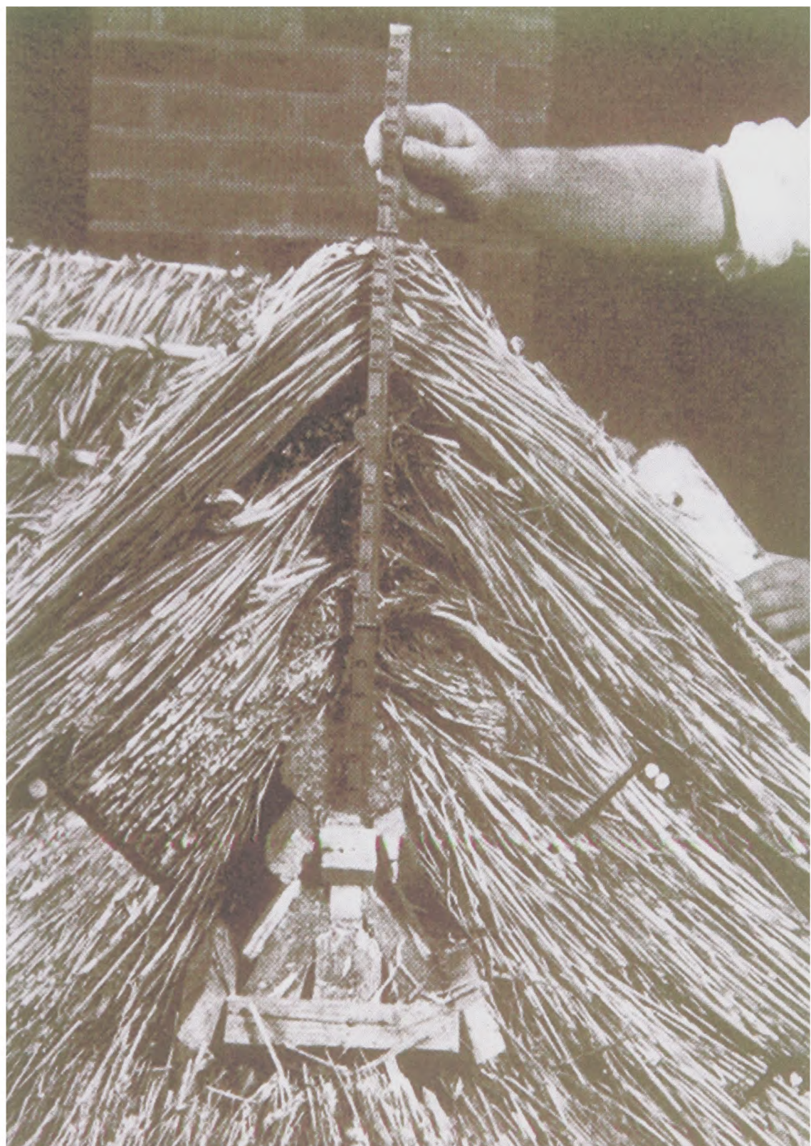
Illustration 54 - The formation of a ridge
