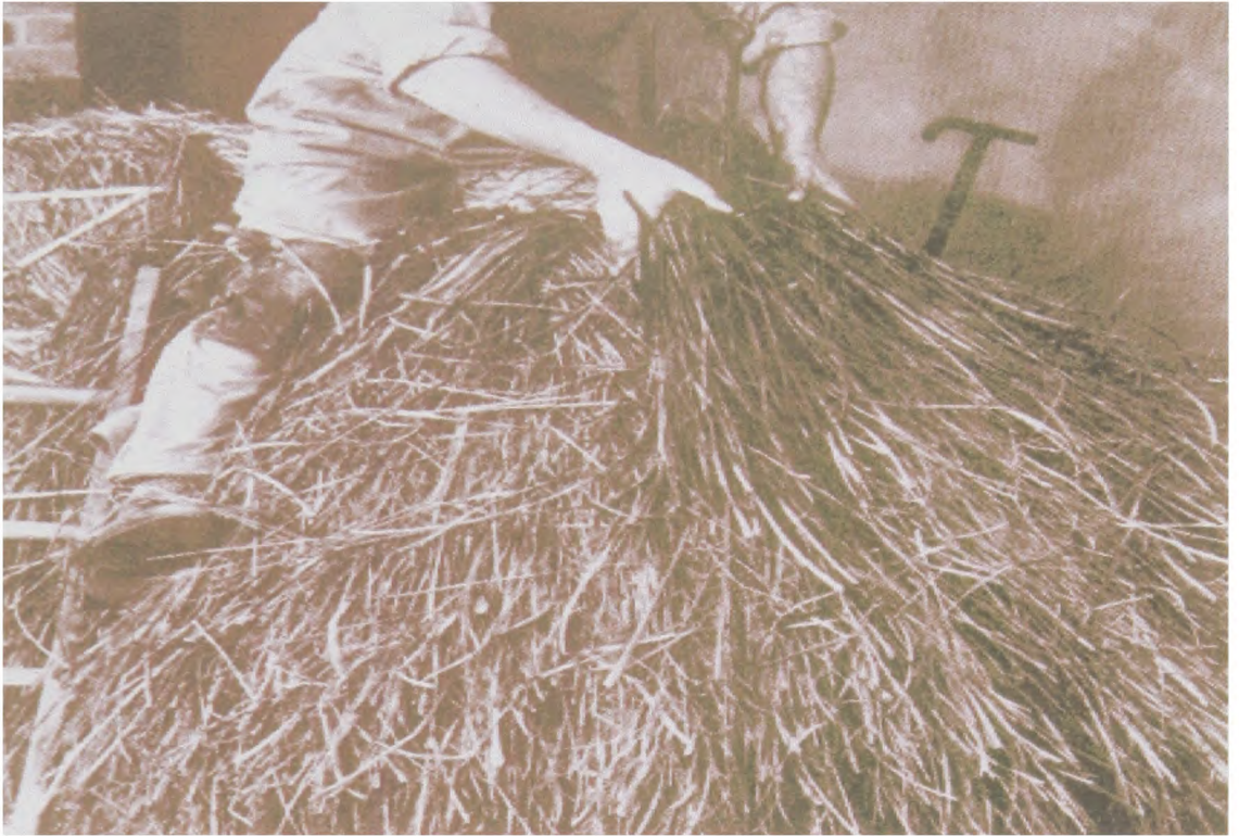
Illustration 43 – A yealm bent round the needle to form a cap end, before it is secured with spars
