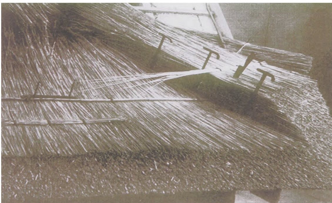
Illustration 63 - The same roof (as in Ill. 62) showing on the extreme right the next course and to its left the temporary sway removed and permanent sways secured into position
