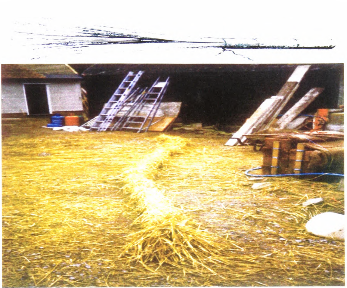
Illustration 23 - Diagram (above) showing how a ridge roll is formed, and (below) a ridge roll before being secured to the roof
