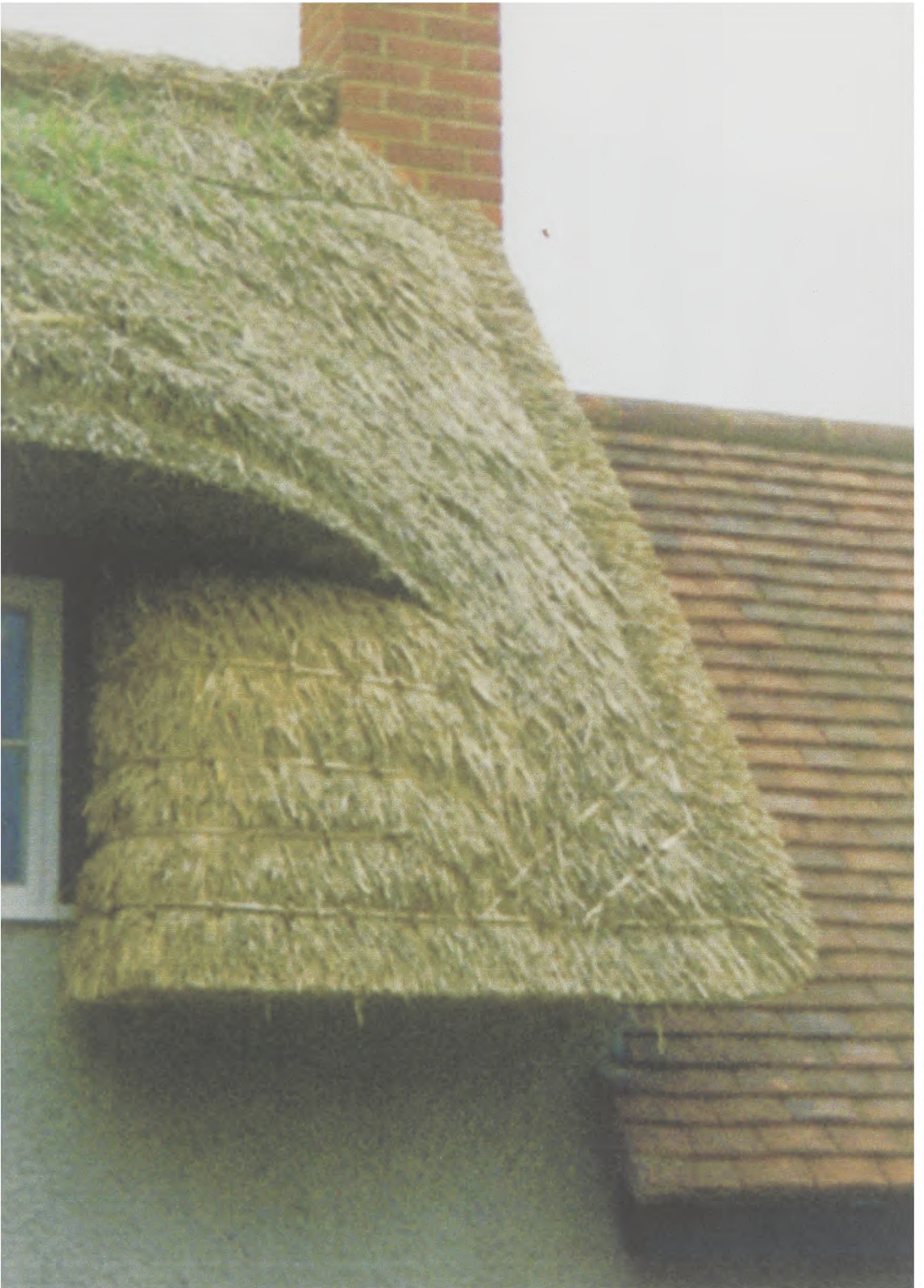
Illustration 8 - Exposed liggers to the eaves and cheek of the eyebrow window at 41 Whitecroft Road, Meldreth (Me 02)
