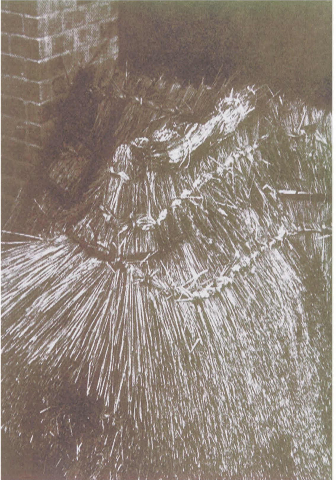
Illustration 55 - A waistcoat layer
