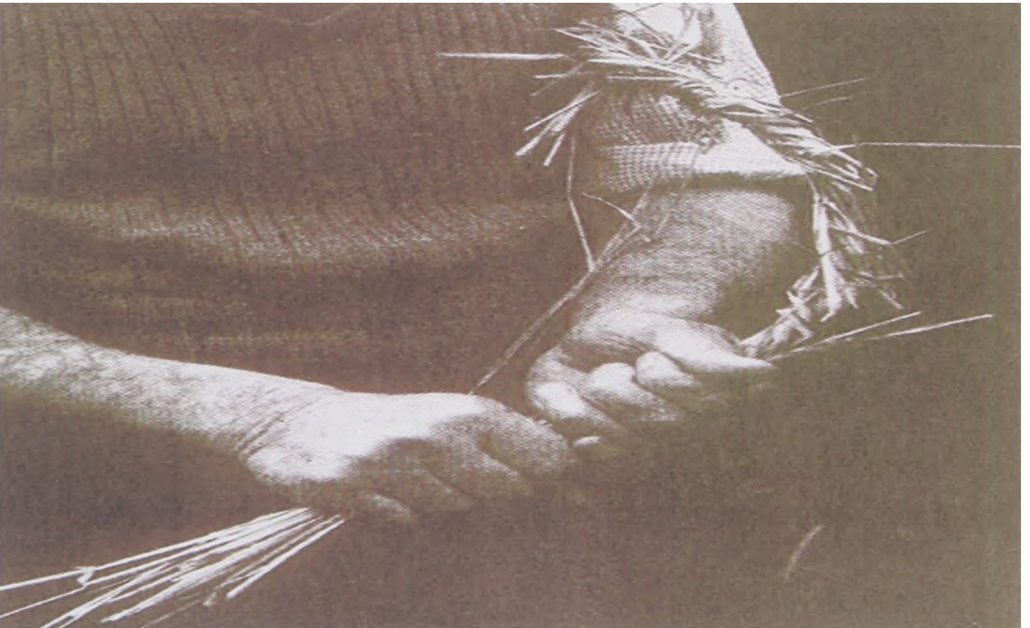
Illustration 26 - A long wheat straw bond being formed
