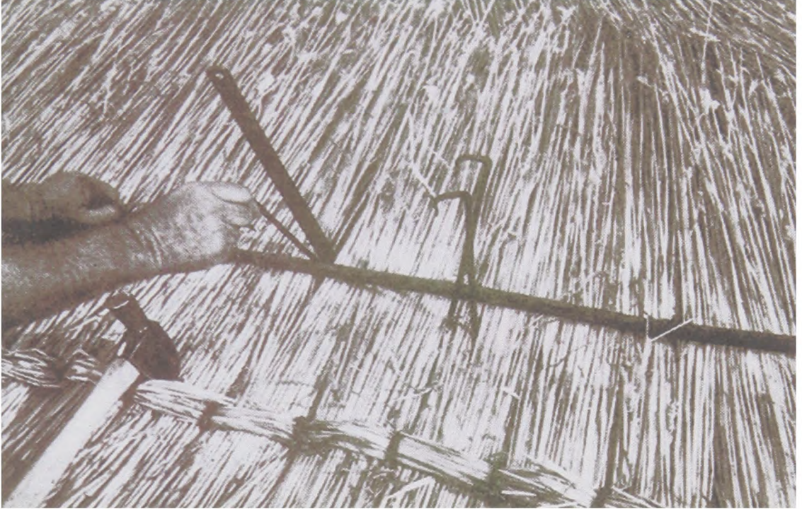
Illustration 51 - A hook about to be hammered into a rafter, located by the needle, to secure the sway shown to its left
