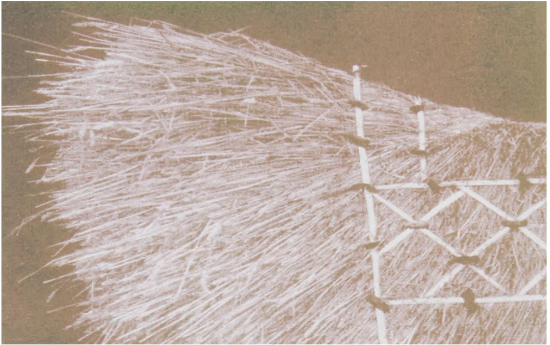
Illustration 45 – The same gable (as in Ill. 44) with yealms packed under the crossed-over liggers
