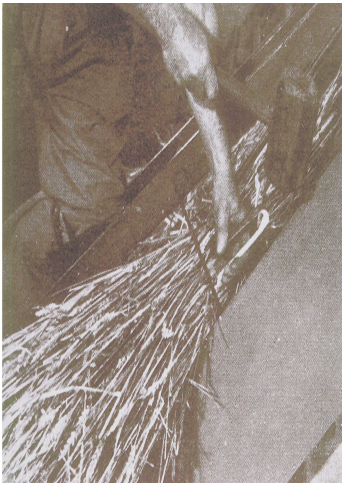
Illustration 33 – An additional spar fixing to the barge bottle
