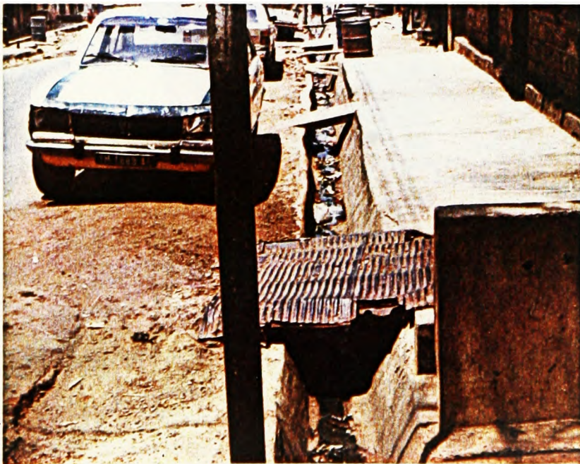
b. Poor Drainage and Sanitation System in the Non-Reservation Layout in Enugu.
