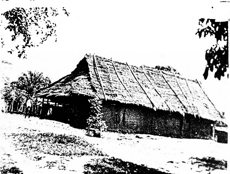
b. Completed Roof.
