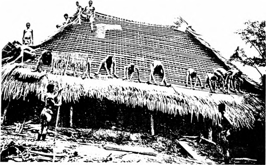
a. Roof Construction in Progress. (after Basden, 1921).
