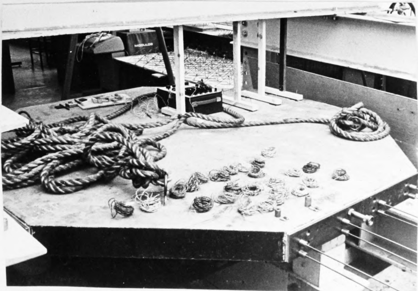
Photograph ( 7.5 ) Fully cast and prestressed slab
