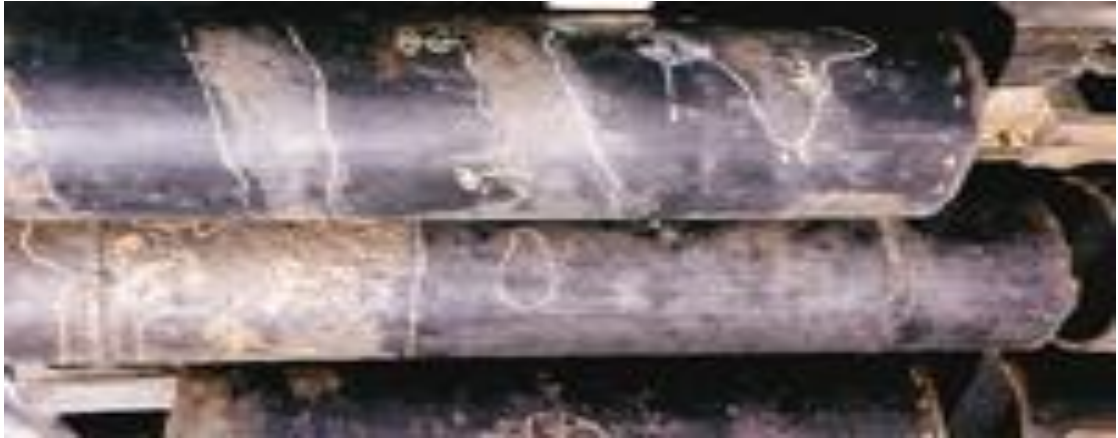
Photo 2.2: Corrosion is Shown Beneath Detached Steel Pipe Coatings
