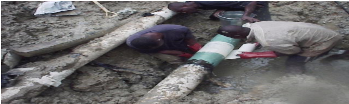
Photo 2.1: Repair and Rehabilitation of Pipeline Facilities (Source: ACT-COSMI)
