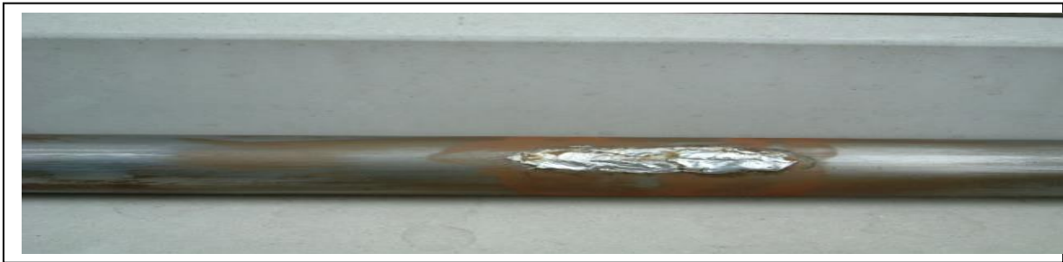
Photo 5.2: The Pipeline System Showing the Sealed Holes
