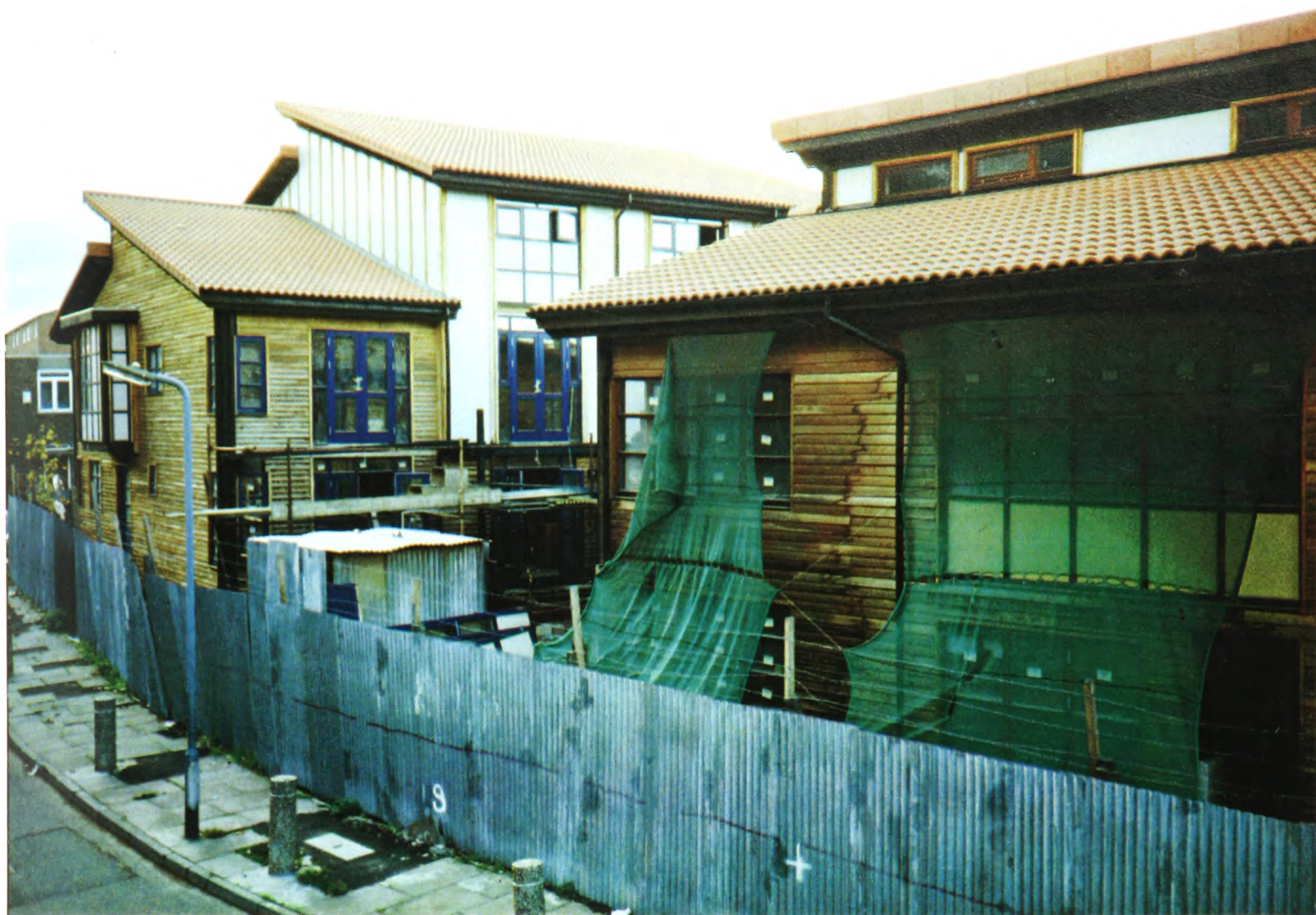
Figure 24 and 25 Two and three storey houses
