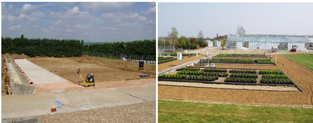
Figure 46. The construction phase of EMWC (left), showing the main central culvert (left edge of image) where drainage water was to be collected and the EMWC in experimental operation with plant material on the different irrigation beds (right).
