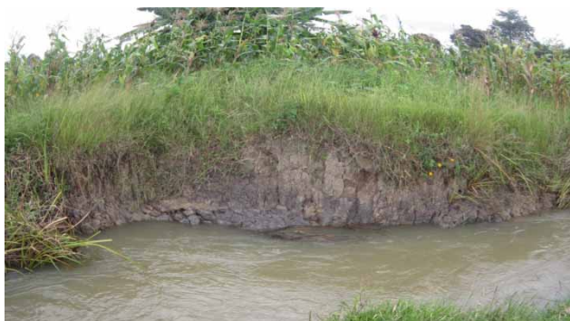
Figure 10 | Eroded Lyandembera Riverbank in Ifunda village. Note the maize field in the background.
