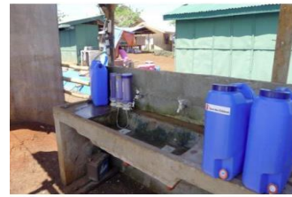
Figure 9(a). Illustration of greywater collection in jerrycans from laundry to be reused for irrigation in the camps (Source: Spuhler, 2012 as cited by Zech et al., 2016).
