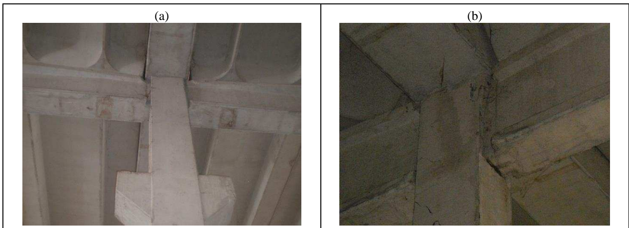
Fig. 8 Damage of the beam-to-column connections after the event on May 29 th
