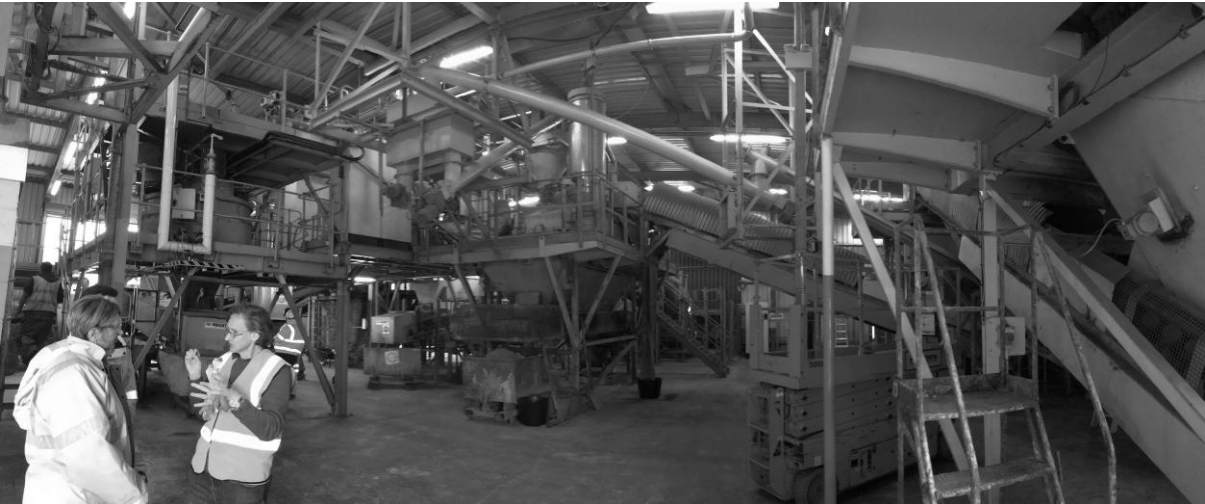
Figure 1. APCr processing plant (second phase)
