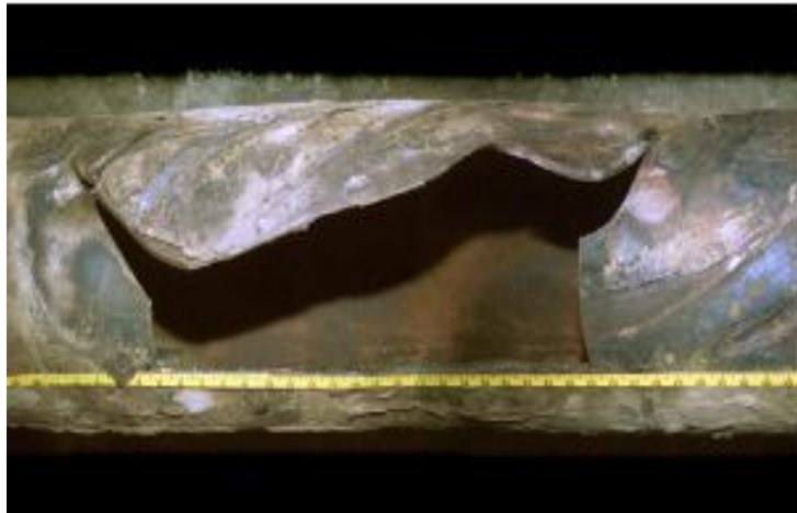
Figure 1.2: A typical pipe failure due to external loadings
