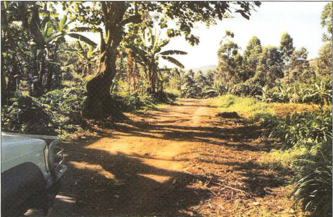
Road in Kasese District. Most roads in Iganga, Kasese and Katakwi District are unsealed, like this one.
