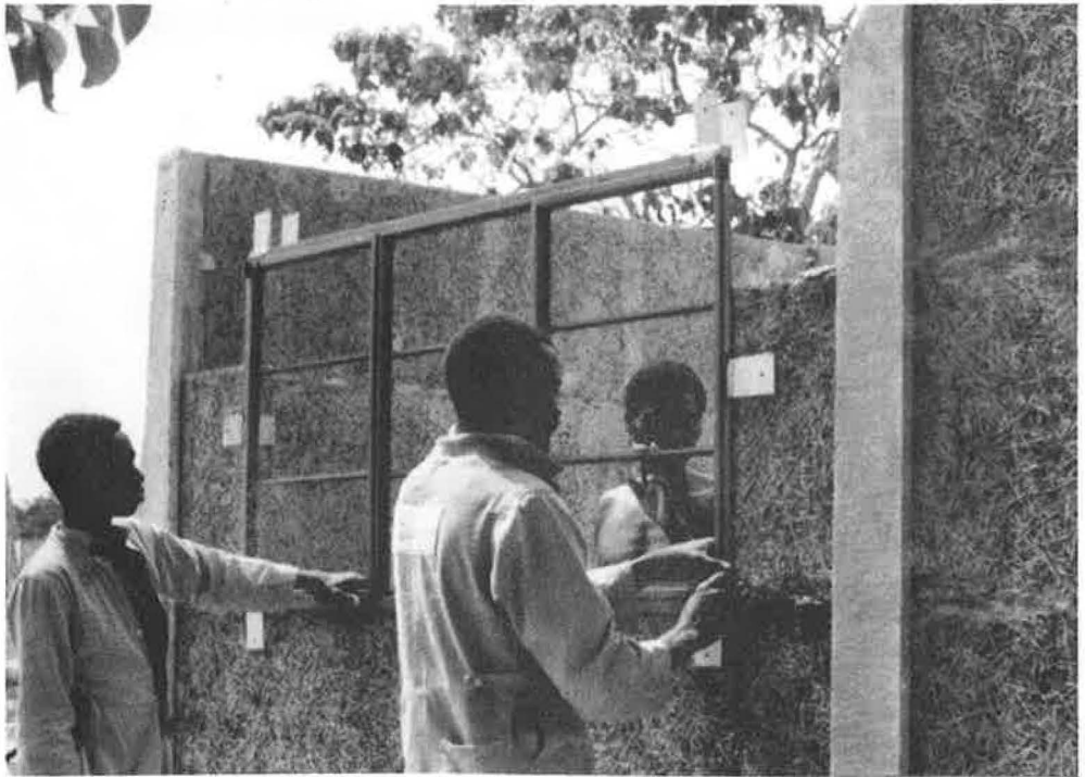
Figure 17 Installing window
