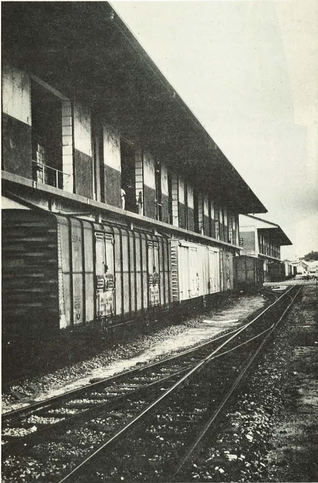
Fig. 1. Types of railtrucks common to East Africa; note the variation in truck size, types of construction and doors.
